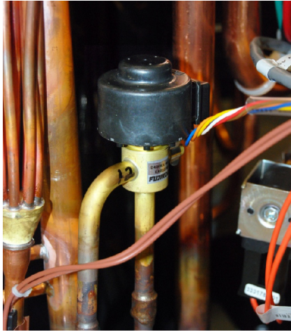
Fig. 2 – Electronic Expansion Valve (EXV)
