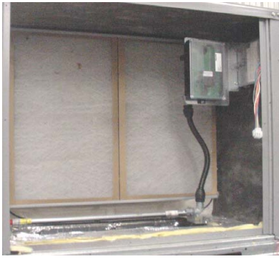
Fig. 23 – Return Air Sensor Operating Position
