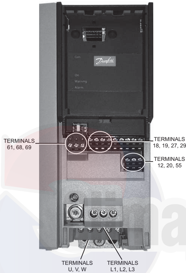
Fig. 38 - Variable Frequency Drive (VFD) Terminals and Connections - unit shown with front cover removed
