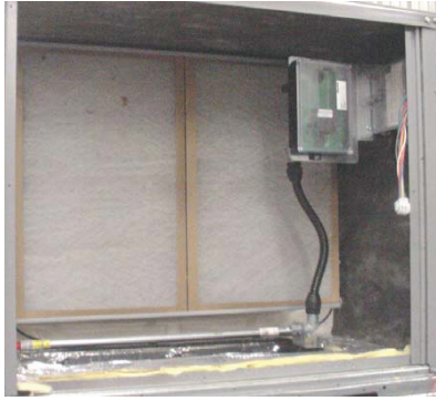
Fig. 41 - Return Air Sensor Operating Position
