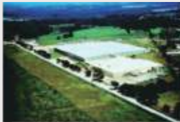
McQuay Auburn Factory, USA
