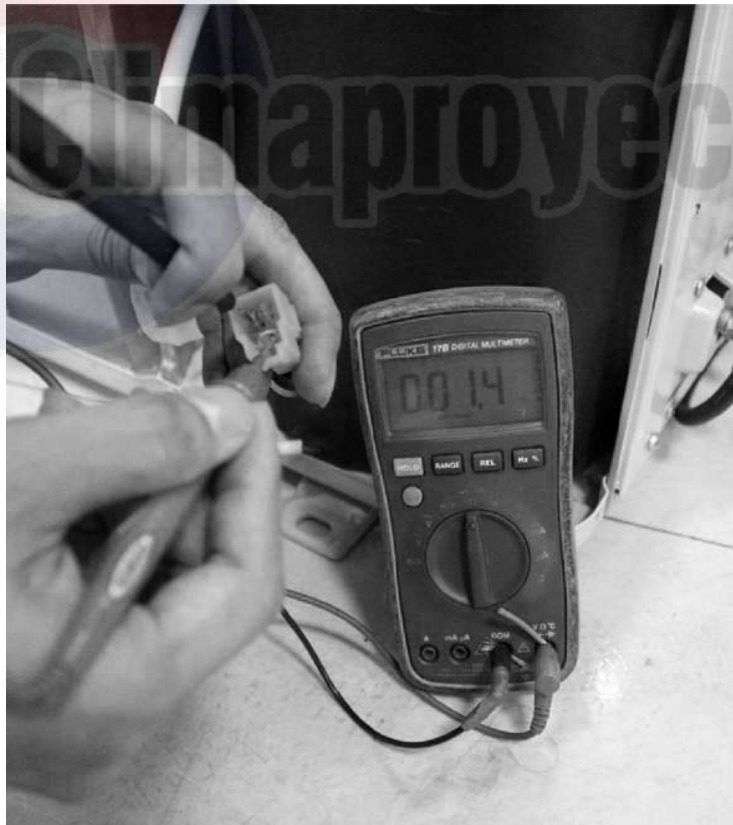
Fig. 27 – Compressor Checking
